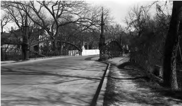
1930s: The Johnson Street Bridge, which crosses the San Antonio River in the King William neighborhood 1
