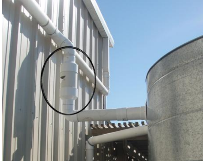
Figure 2. Self-cleaning filter for tree litter and similarly sized particulates
