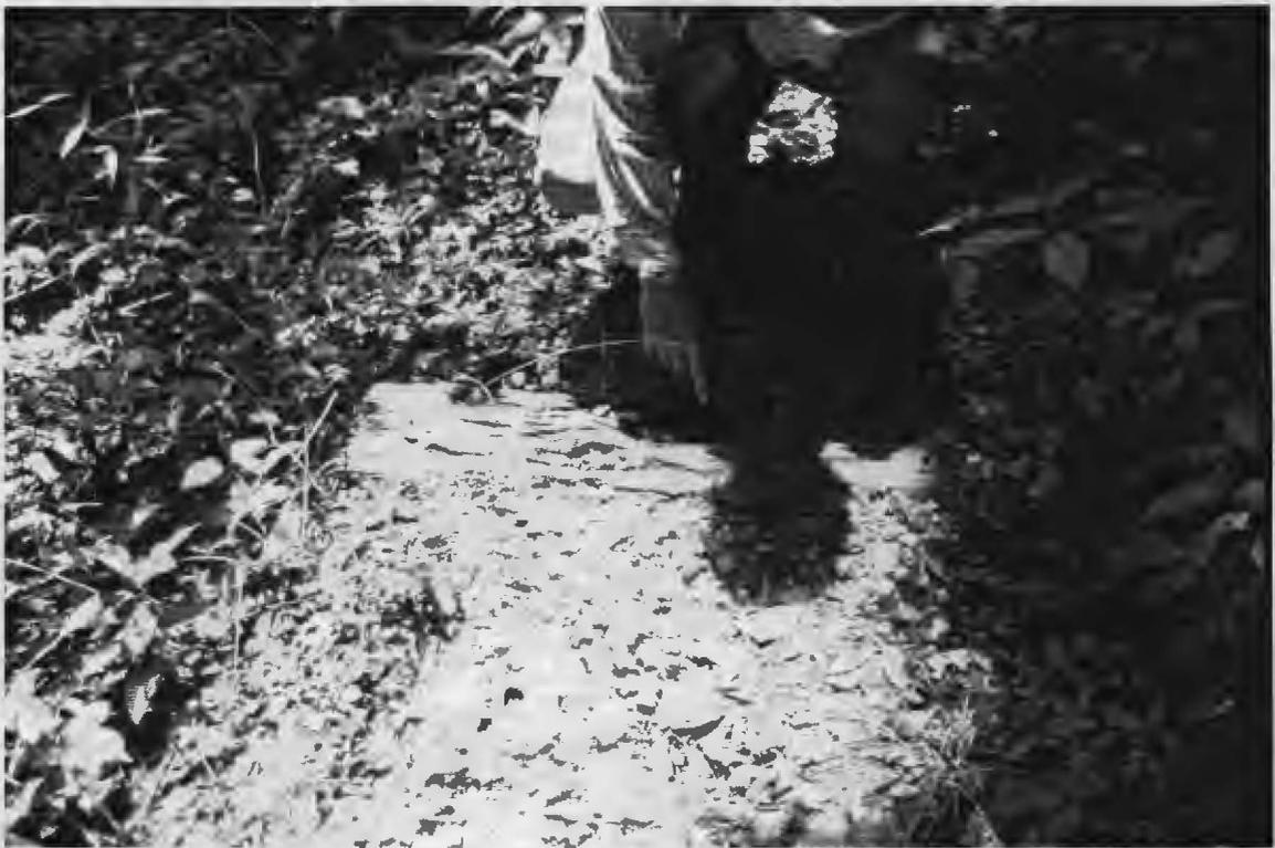
Figure 9.5. Roughly hewn railroad ties laid in gravel on top of a wider (4 m) road bed.
